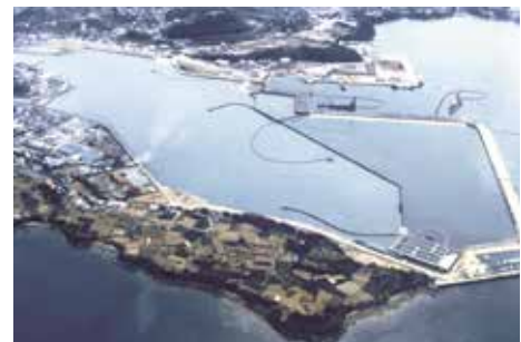
Dredging using a Cutterless Pump Dredging Ship
