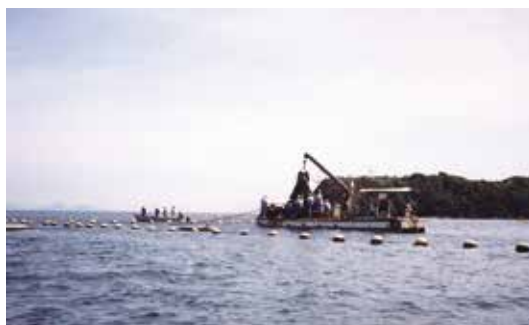
Removal of the Dividing Nets
